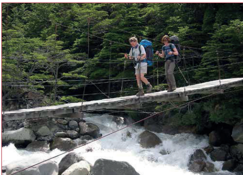
FIGURE 7.25 TYPICAL SUSPENSION BRIDGE CROSSING IN TORRES DEL PAINE
