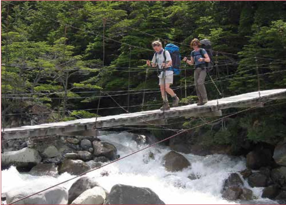
FIGURE 7.25 TYPICAL SUSPENSION BRIDGE CROSSING IN TORRES DEL PAINE Photo: Helen Barnard
